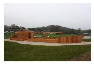
The barge was fitted in accordance with the manufacturer's detailed plans and instalment instructions. The ground underneath was layered with a geotextile membrane, followed by clean stones, which allows water to collect and slowly soak away, and then the sand was laid.
