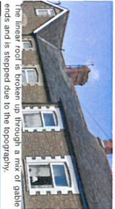
Crag tile roof with brick chimney, hipped away from the street but at varying heights within the terrace.
