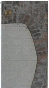
Traditional stone detailing to the garage door
