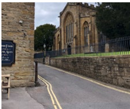
7. The low wall defines a clear boundary whilst offering views to the Minster and green space behind.
