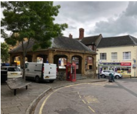
1. Poorly placed street furniture, and road signage creates clutter obscuring historic features.
