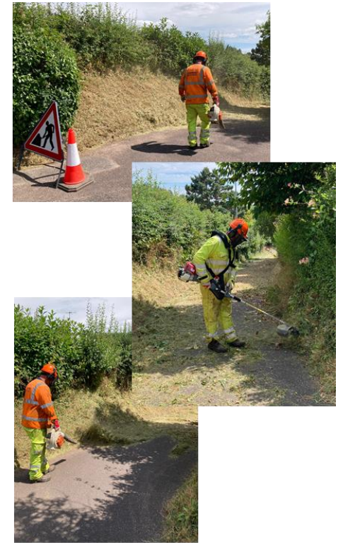
Works get underway
