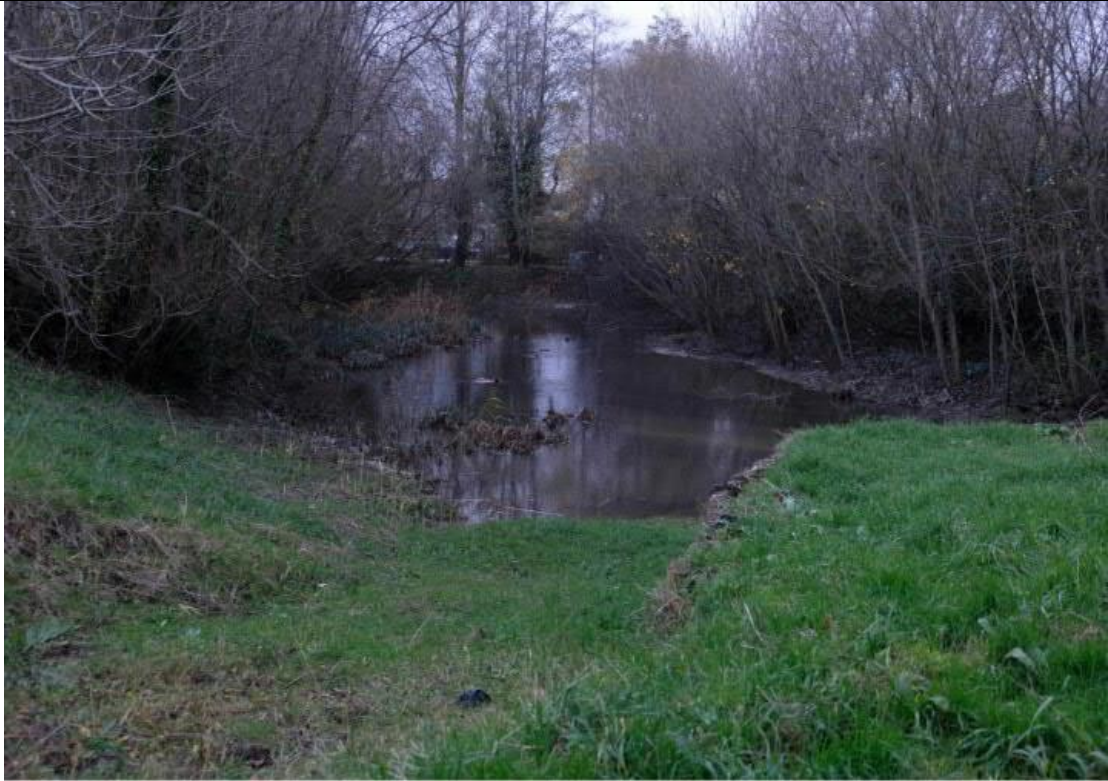
Figure 12: Storage area near Station Road. (Taken after flood waters had subsided)
