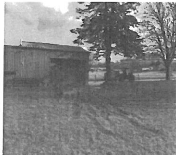
Looking towards Wardens' workshop
