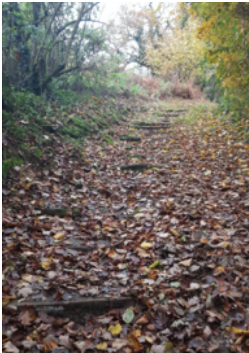
Old steps to be replaced due to weathering and erosion.
