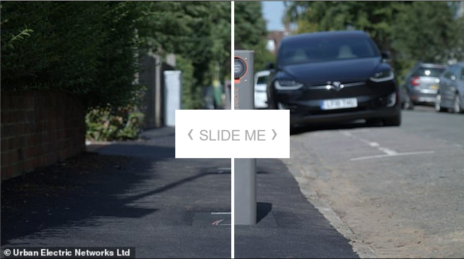
Pop-up power: These are the UK's first retractable street chargers that rise out of the ground. They've been installed in residential streets in Oxford (pictured) and Dundee
